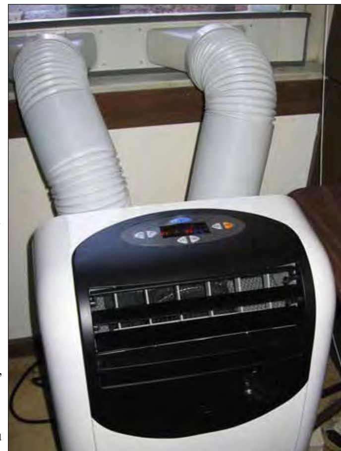
This Soleus portable heat pump can be attached to any window to provide efficient heating for that room.
