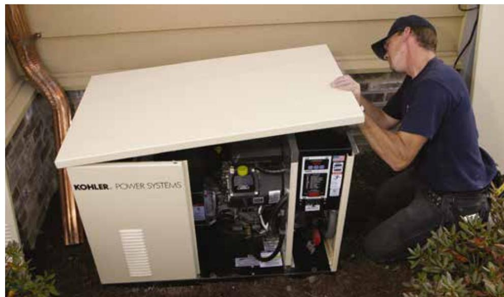
**ABOVE:** This is a whole-house sized standby generator being installed at a home. Notice the small gas engine inside the housing. **RIGHT:** This shows the typical electrical connect from a standby generator to the house wiring.
