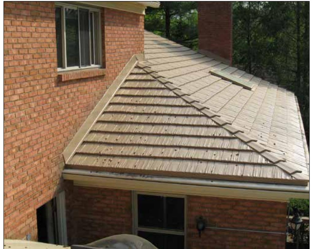
**ABOVE:** The completed metal roofing with new flashing and decorative hip trim over the seam. **BELOW:** The metal roofing panels are being installed over the underlayment. Hidden stainless steel nails and aluminum clips are used to secure each panel.
