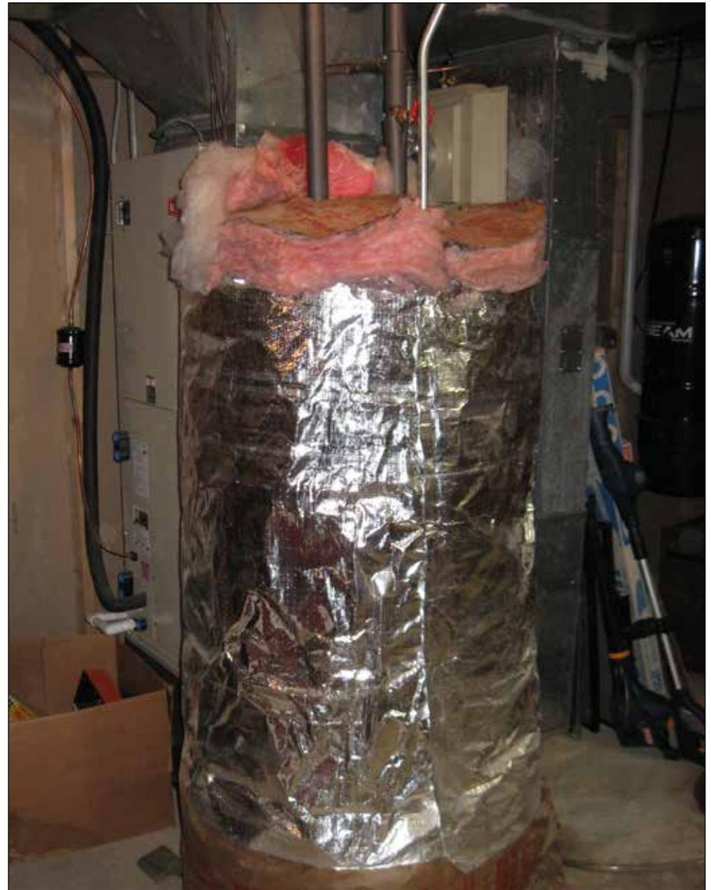
**This tall 80-gallon electric water heater is first wrapped with fiberglass insulation and then with construction foil to block radiant heat loss.**
