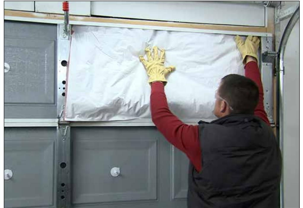
**ABOVE:** After clips are stuck to garage door, the fiberglass batts are pressed over the clips. **BELOW LEFT:** This garage door panel has polyurethane foam insulation and interlocking seals between the panels to minimize air leakage.
