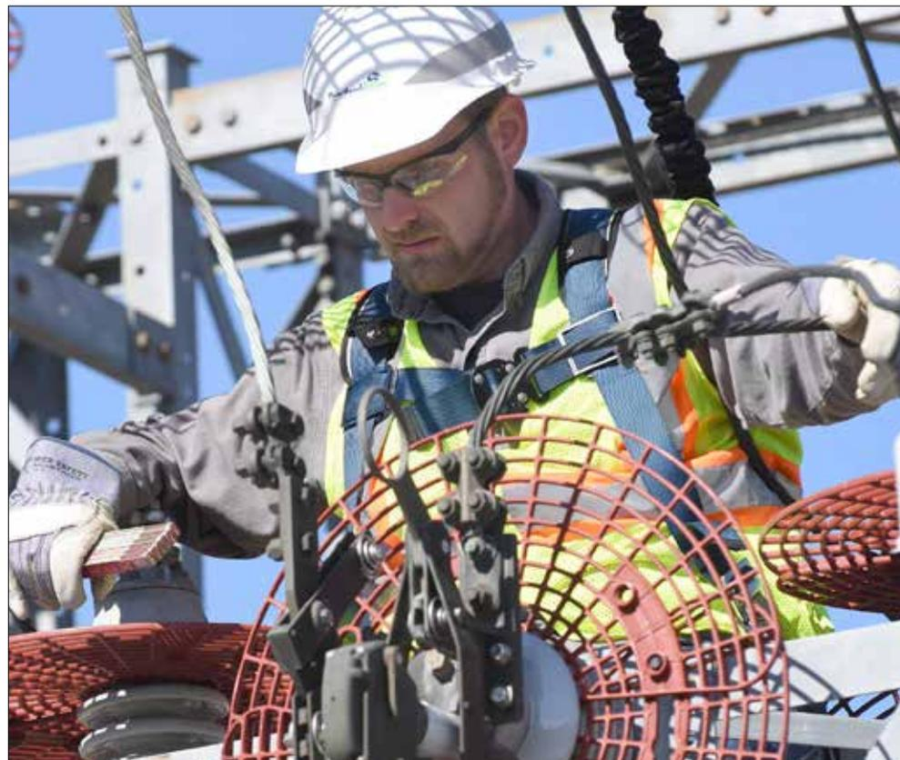
**Heartland crews, including Ryan Stifter here, were working at our Hiattville substation recently to install coverup. The dark red protective coverup helps keep birds, snakes, and other animals from making contact with live substation equipment. This reduces outages and helps us keep the power on for our members.**
