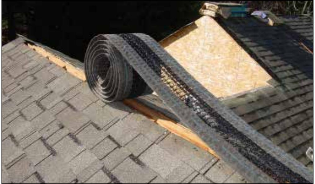
**A mesh low-profile ridge vent is barely perceptible from the ground. The mesh vent is rolled out, laid smooth, and cut to length. After it is attached with a nail gun or hammer, wide shingles are tacked over the top.**
