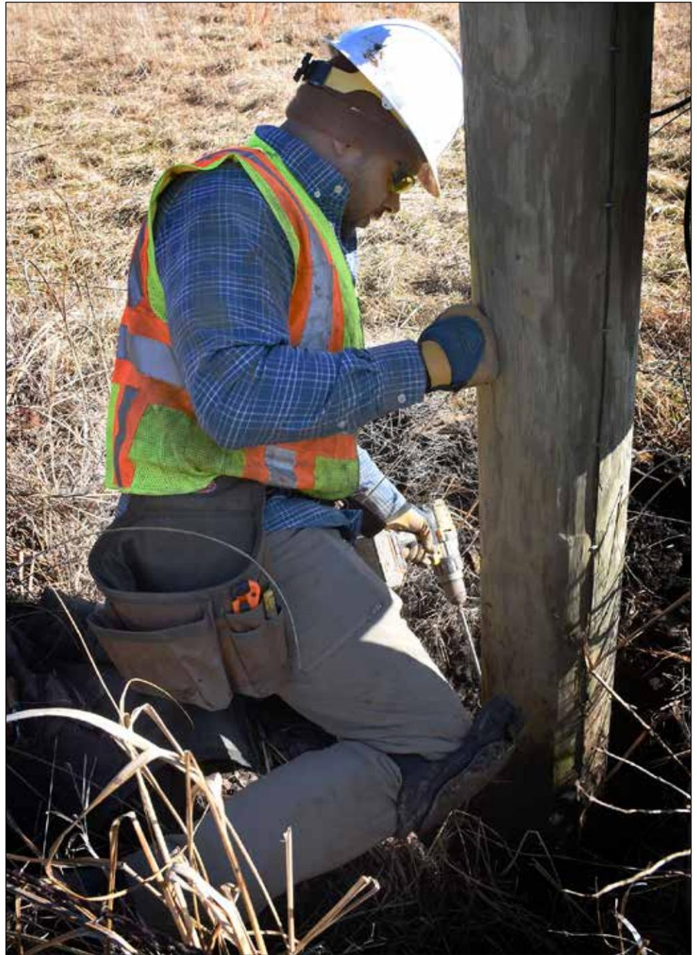
Inspecting, testing, and treating Heartland's utility poles is an annual process, extending the life of the poles, and improving reliability. Heartland partners with a company, Osmose, to inspect the poles and help recommend pole replacements when needed.
