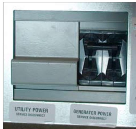
**During an outage, the interlock handle should be moved to the left and the "Generator Power" breakers are turned on to allow generator power to flow into the home.**
