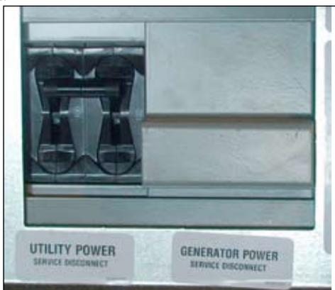
**Under normal conditions, the "Utility Power" breakers, located on the left side of the panel, are up, allowing Heartland's power to flow through the panel.**
