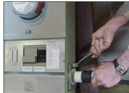
**The power cord connects the generator to the transfer switch.**
