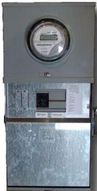
**Removing the protective door gives Heartland members access to the breakers that control the flow of power from HREC and a standby generator.**
